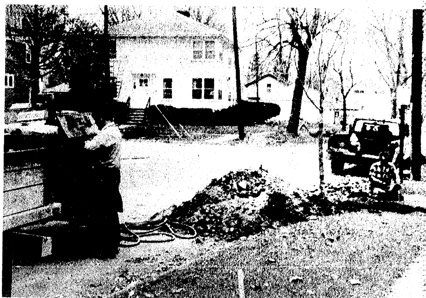
GAS COMPANY AT WORK: Crews of Michigan Consolidated Gas Co. have been working along Madison St. between Middle and Park Sts. for the past several days, repairing transmission lines. Traffic has been slowed but not stopped.
